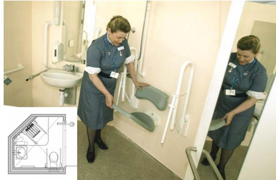
The above example illustrates that en-suite facilities can be provided in the smallest of spaces making a vast improvement to the patient’s experience. The wall opens up to allow access, then closes for privacy.
